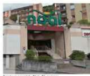
Exterior view of the Noab shopping center in Lunnegiane.
